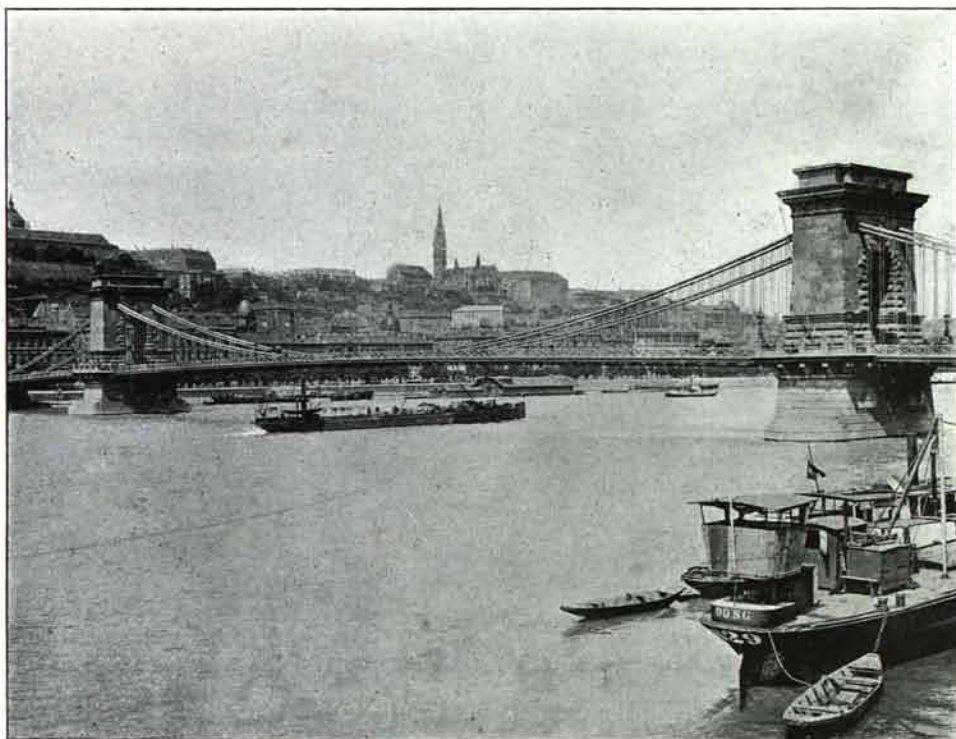
BUDA PESTH.—SUSPENSION BRIDGE.
